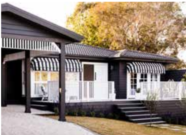
Concrete Elabana in Barramundi
