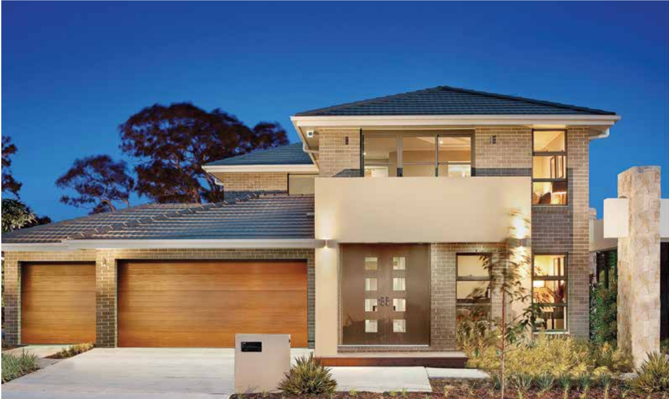
Designer Home featuring Monier Tiles, Concrete Atura in Barramundi
