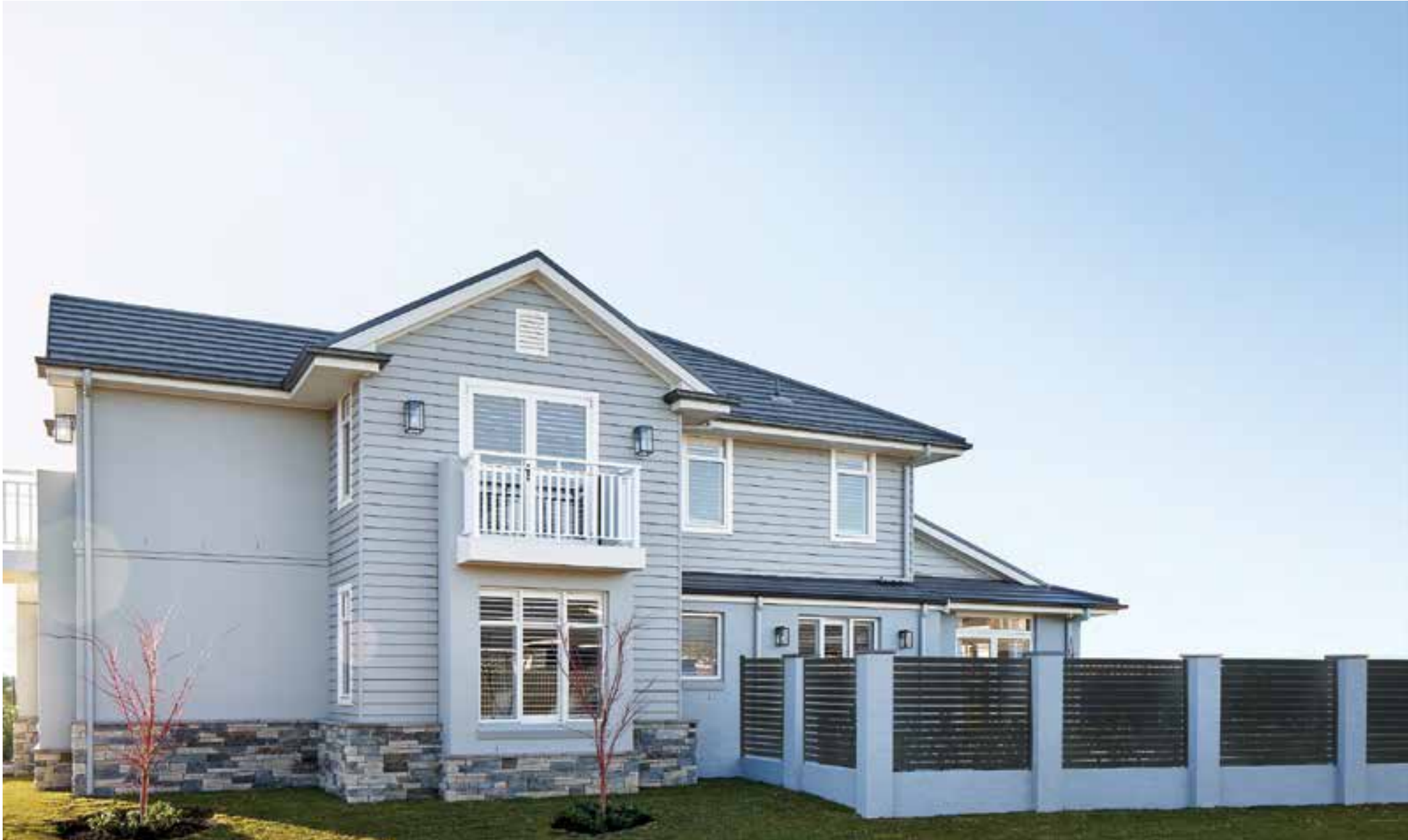
A custom-built Hamptons style home by Masterton Homes featuring Monier Tiles, Concrete Horizon in Barramundi
